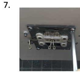
Remount socket. Torque 0.50Nm.
