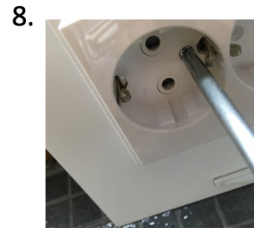
Remount cover by hand. Do not tighten screws excessively.
